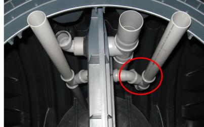
Shorten the overflow baffler at the marking for installation in Graf tanks (see diag. above).
