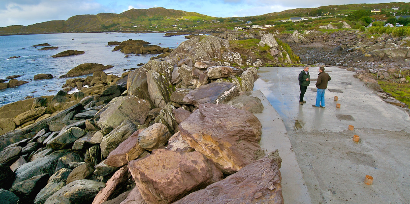
Directly on the water: The Derrynane Hotel wastewater treatment plant lies only a few steps away from the Atlantic. An AQUAMAX® PROFESSIONAL XL-2 250 here ensures optimum treatment of the complete wastewater from the hotel operation. Also on the photo: Wayne Paterson Mundell (left) and Patrick Buckley.
