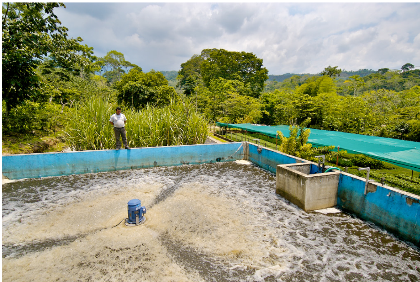
74 % less energy consumption, 74 % less costs: Eliazar Montejo Gonzalez, responsible for the wastewater treatment plant of the finca, observes the new AQUAMAX® PROFESSIONAL XXL-1.
